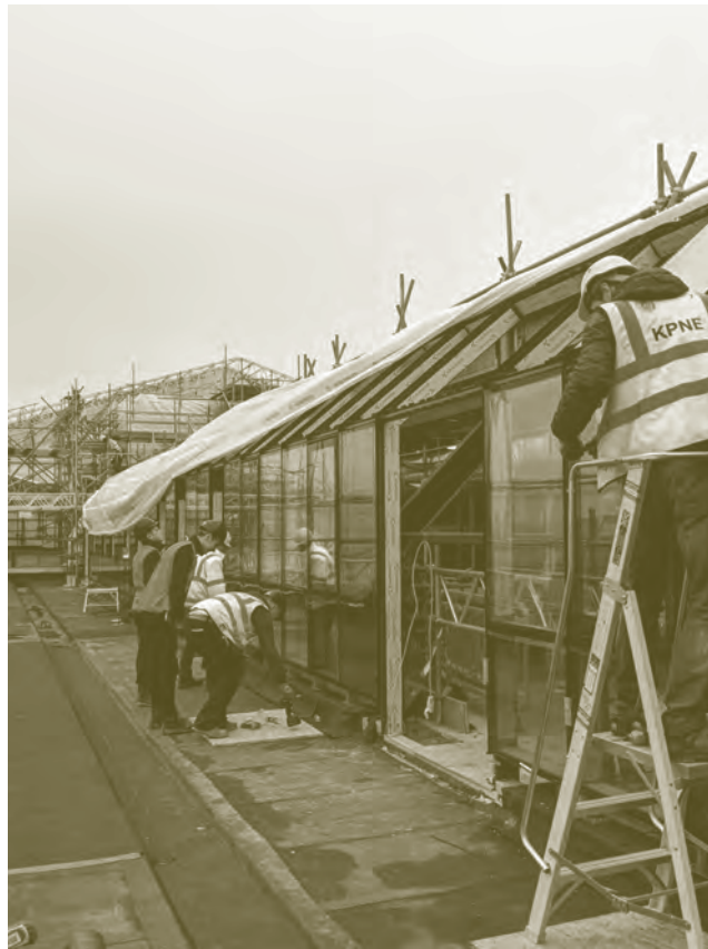
Sloped glazing being installed on studios
