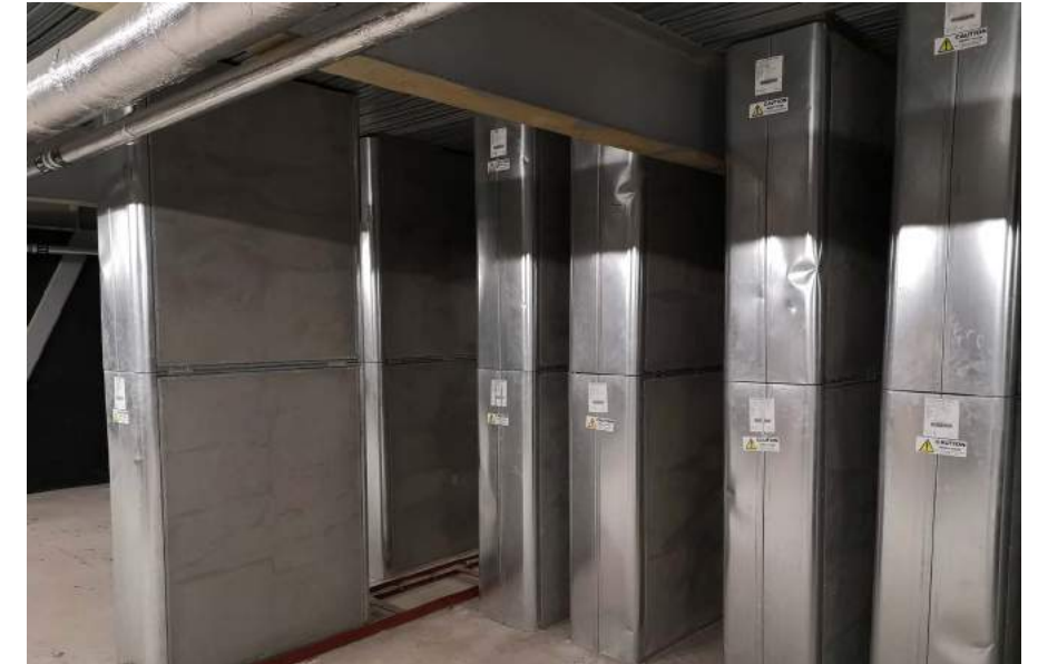
Acoustic attenuators on top floor
