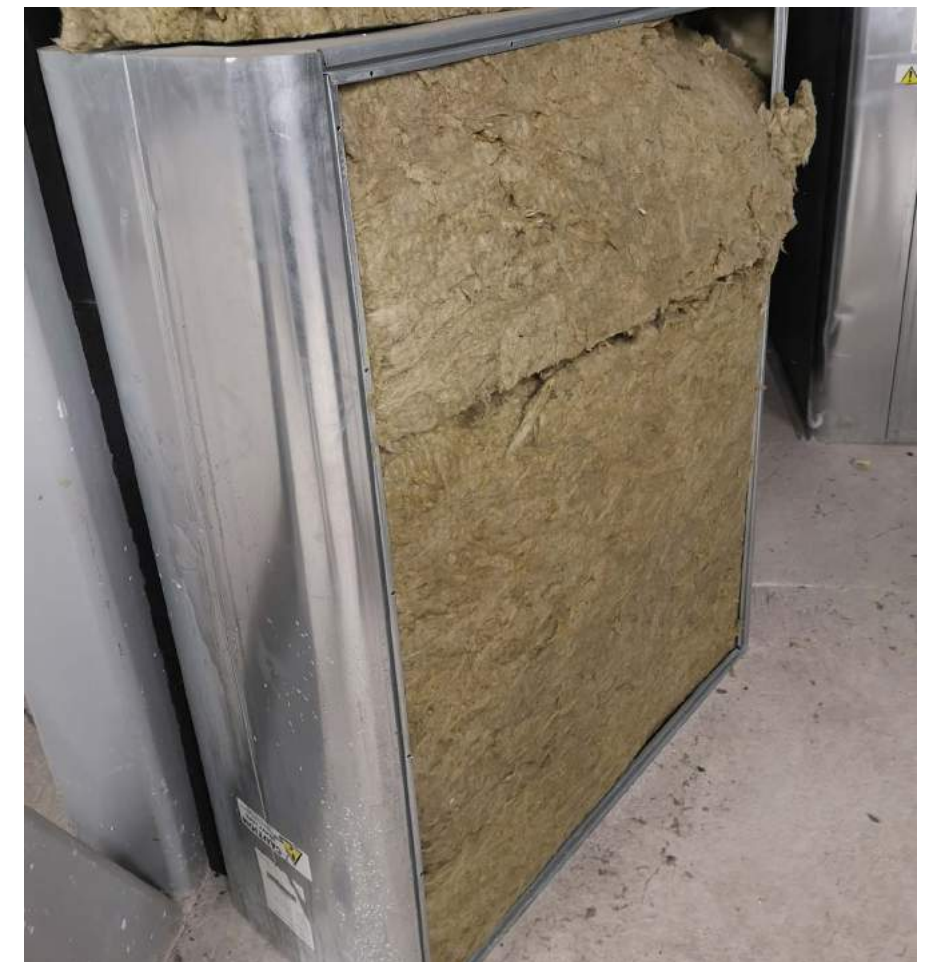
Detail of acoustic attenuator (part of the natural ventilation strategy)
