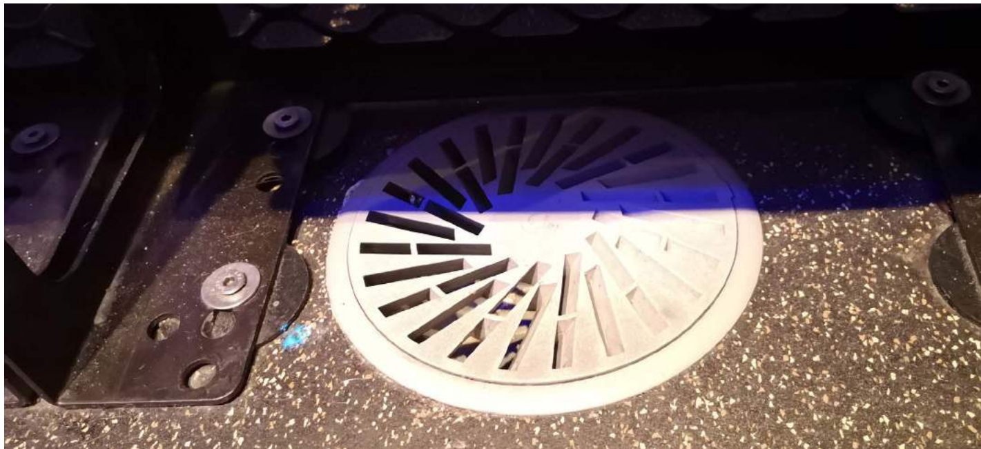
Auditorium - ventilation floor diffuser
