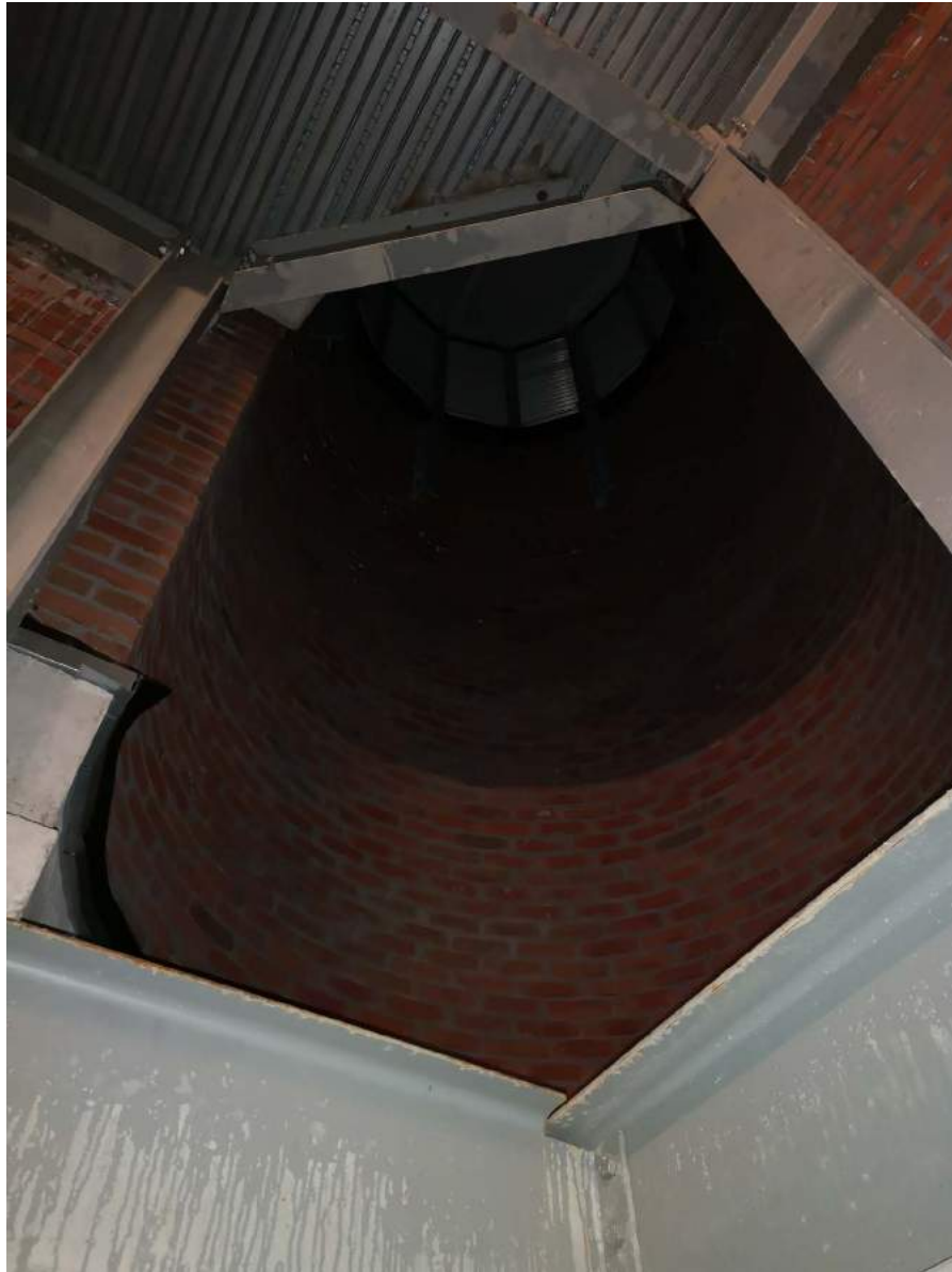
View up to one of the ventilation towers (part of the natural ventilation strategy)
