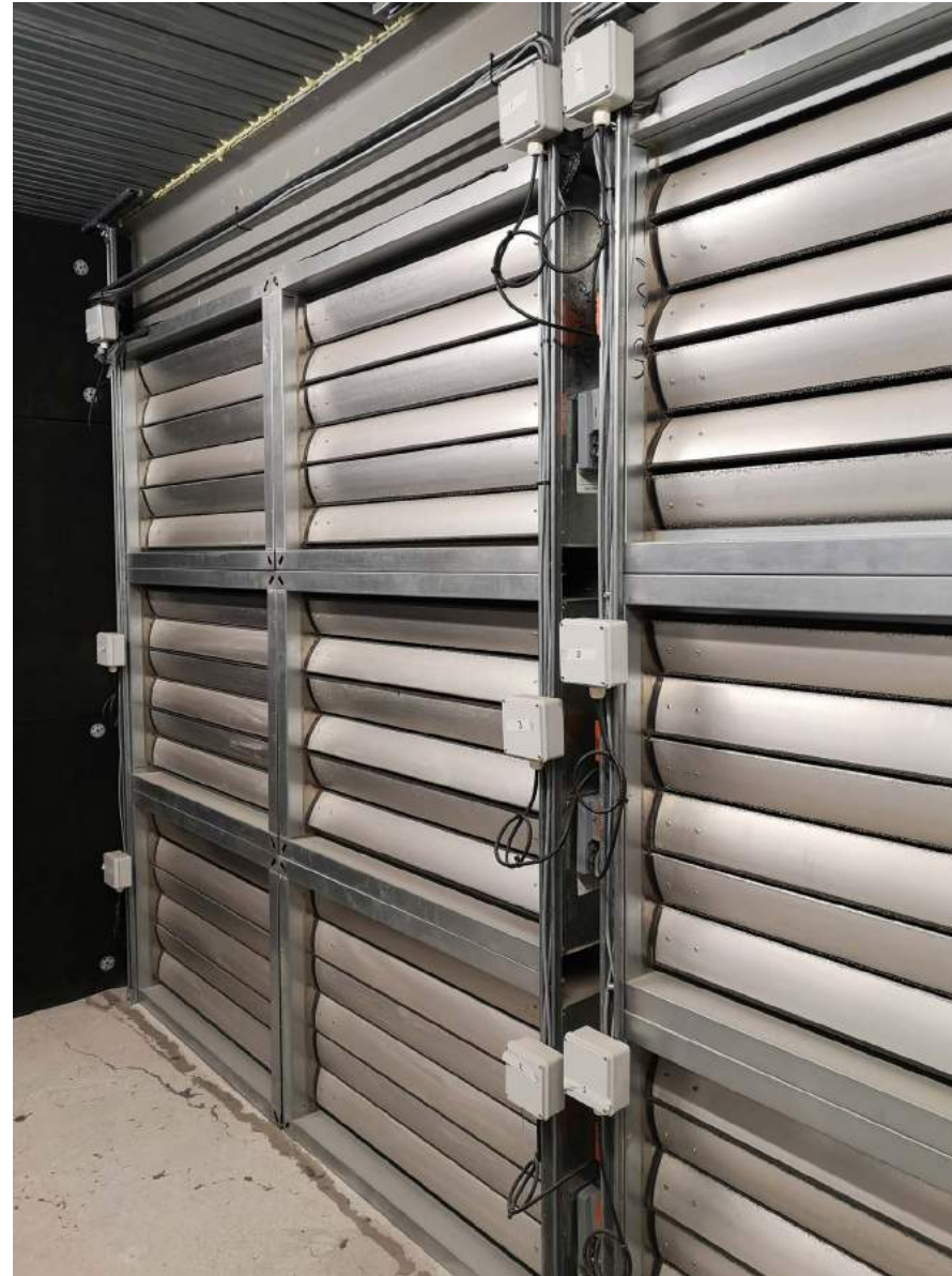
Motorised louvres at top of building (part of the natural ventilation strategy)
